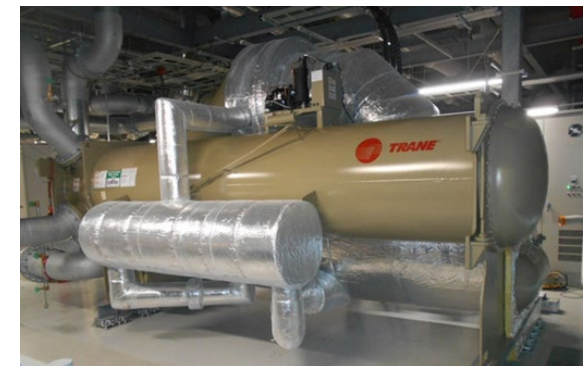
Centrifugal chiller with Non-Freon refrigerant
