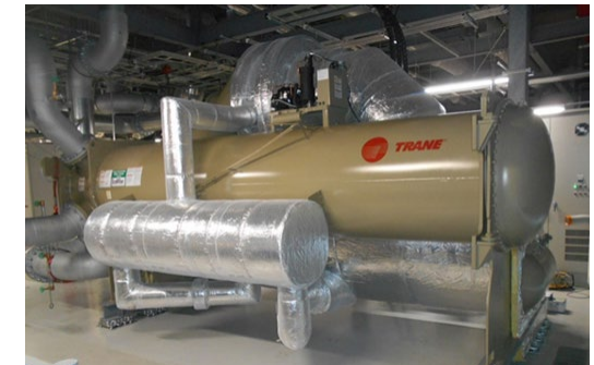
Centrifugal chiller with Non-Freon refrigerant
